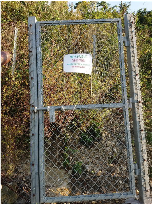
Photo 2 – Current situation of fencing and warning sign
